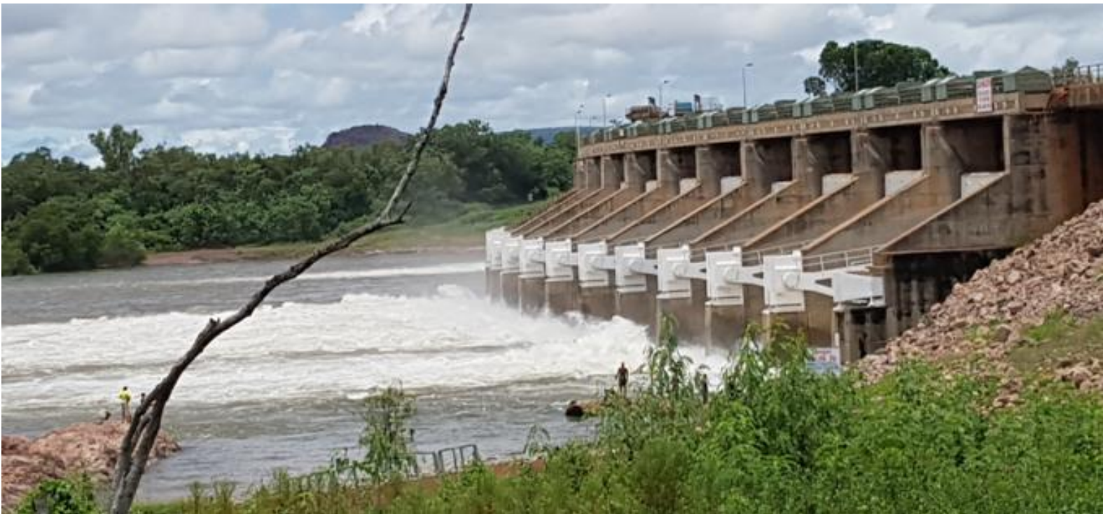
Image 5: Kununurra Diversion Dam
