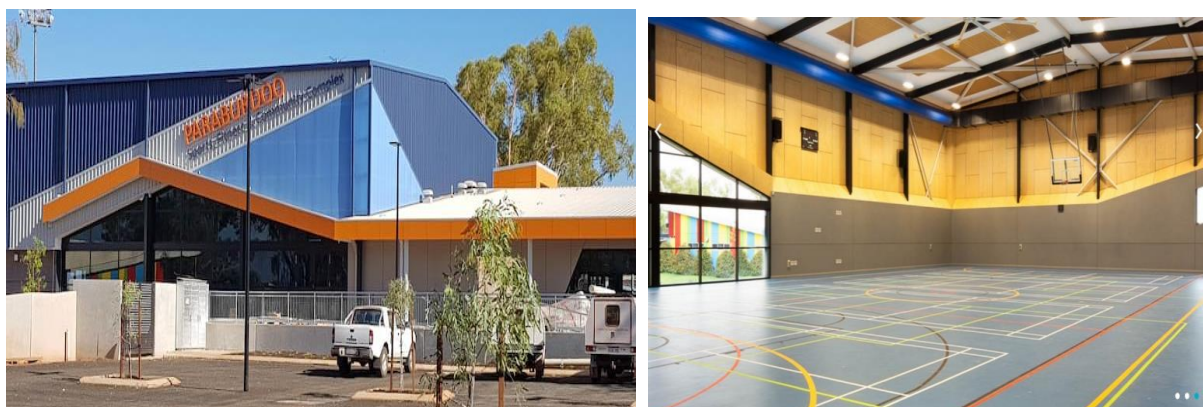
Paraburdoo Sports, Fitness and Community Complex – showing the new construction combined with the existing building
