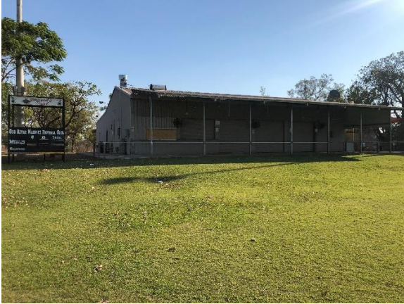
Photo 1- Front View of Club House
