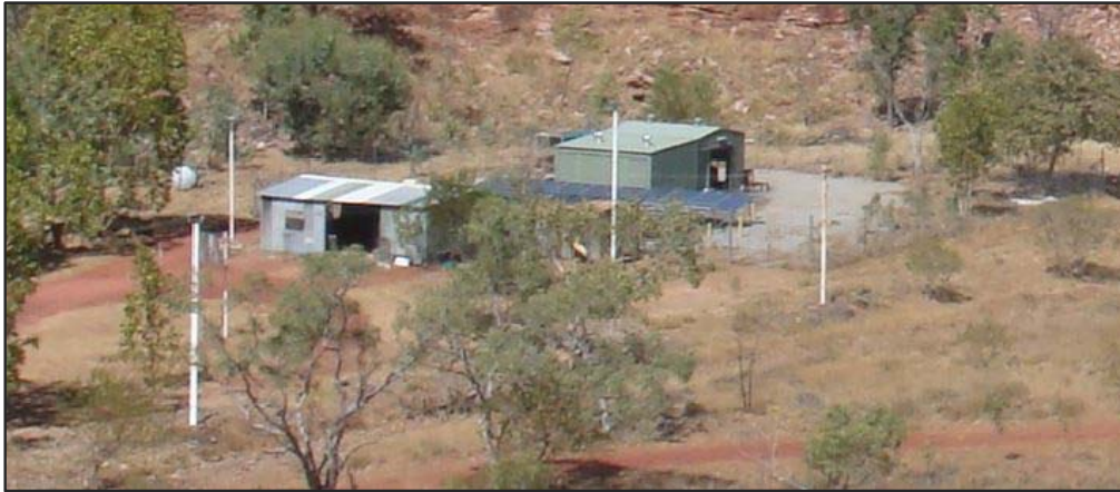
Figure 3 – Generator sheds and solar panel array (2008)
