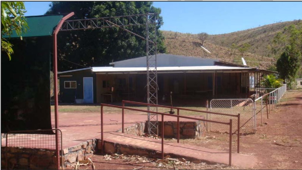
Figure 4 – Community store and stage (2008)
