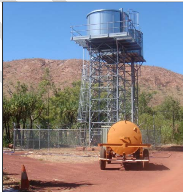
Figure 3 – Elevated water tanks (2008)
