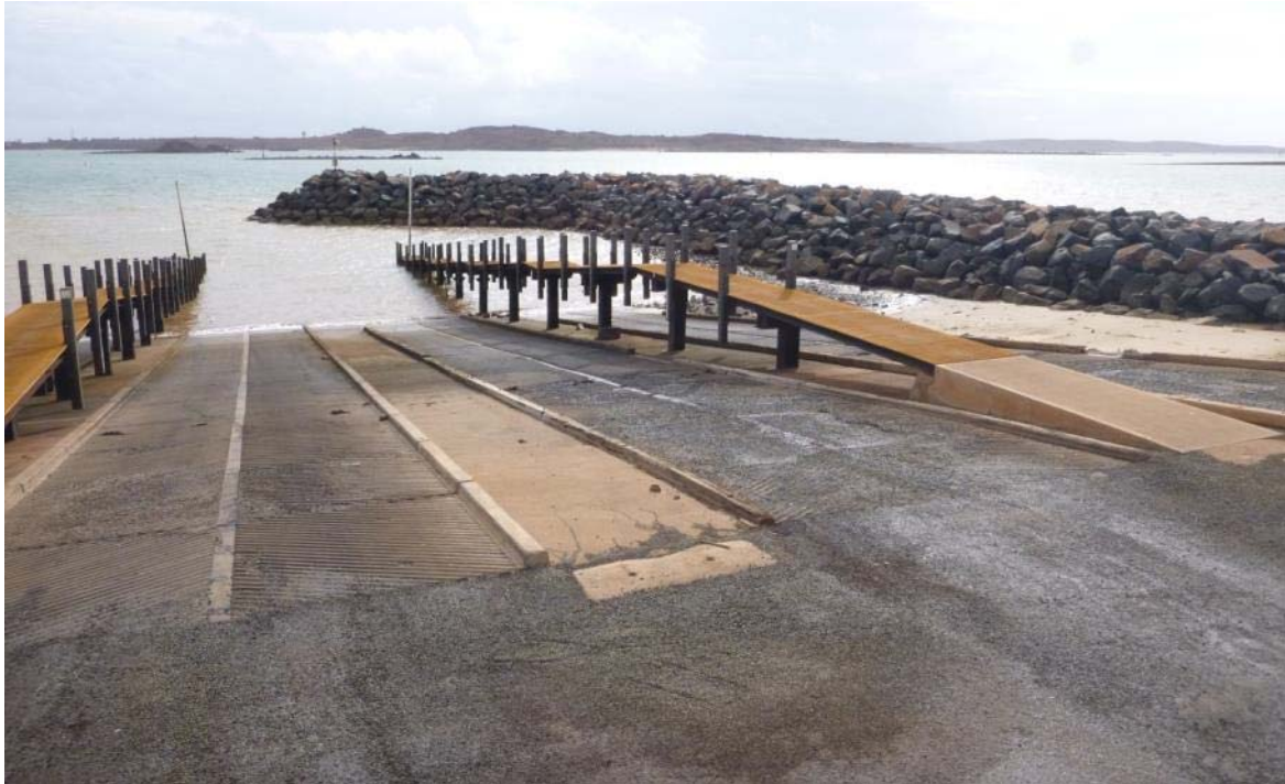
Figure 6-8 Example of a fixed sloping low level jetty (Dampier boat ramp)
