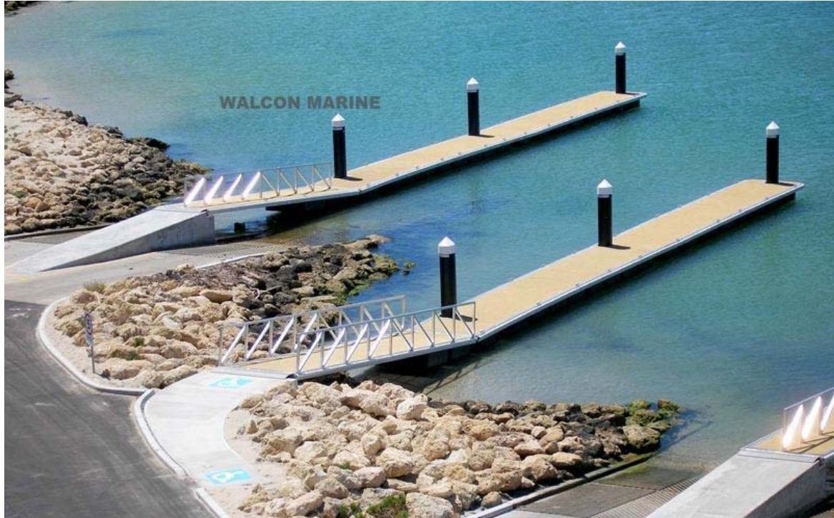
Figure 6-7 Typical Proprietary Floating Pontoon (Ref. Walcon Marine)
