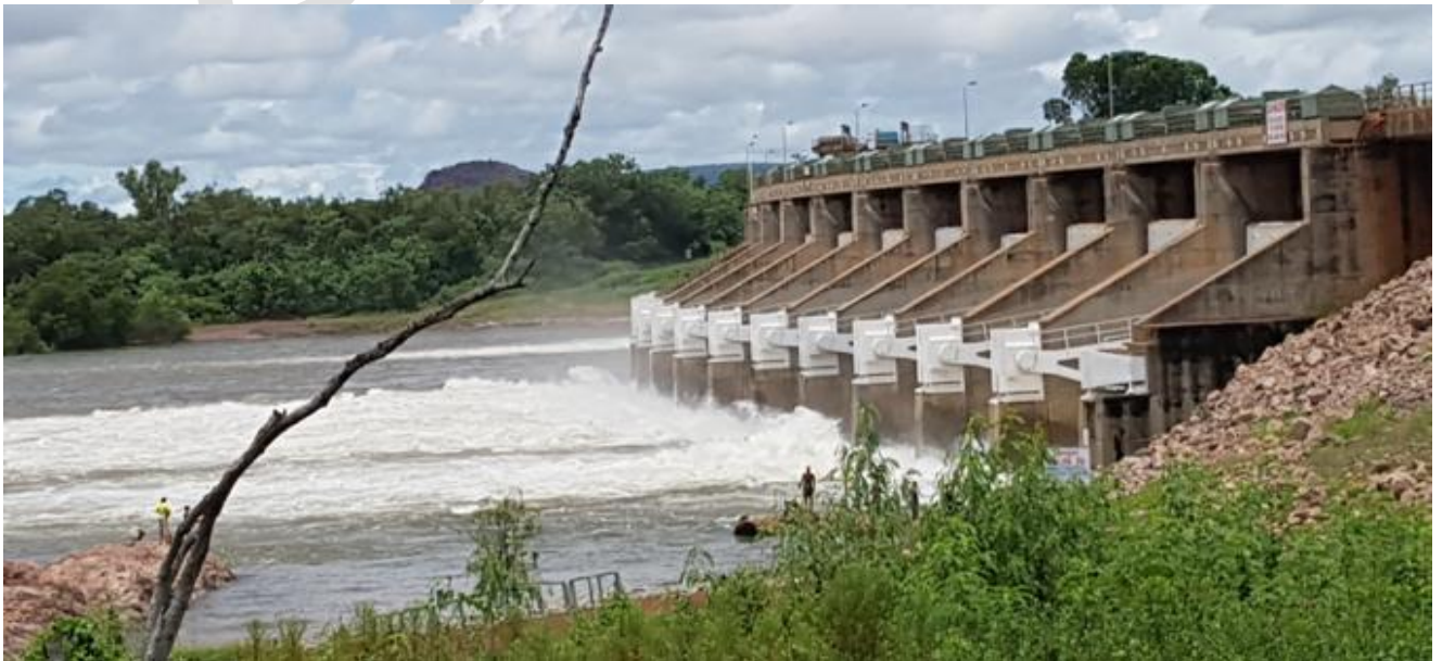
Image 5: Kununurra Diversion Dam
