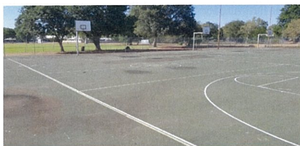
Ponding and surface deterioration
