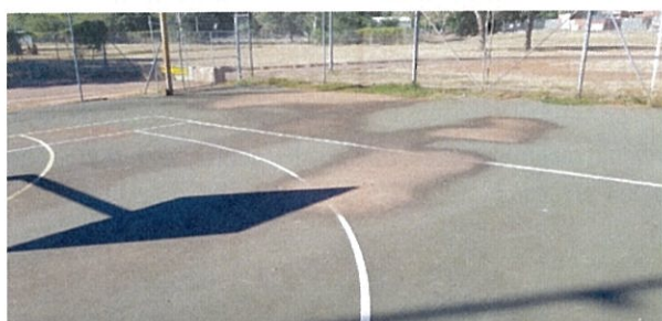
Ponding and surface deterioration
