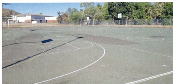
Ponding and surface deterioration
