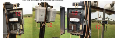
LIGHT TOWER 13 - Both sides of tower working fine New earth required and cables re terminated
