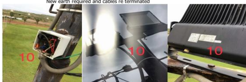
LIGHT TOWER 10 Left side - working fine LED Right side - faulty LED fitting New earth required and cables re terminated
