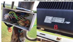
LIGHT TOWER 9 - LED lights both sides working fine New earth required and cables re terminated
