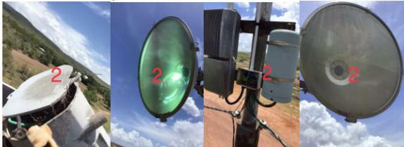
LIGHT TOWER 3 left light - faulty globe Right light - faulty ballast and globe New earth required and cables re terminated
