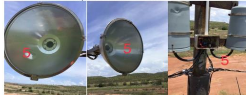
LIGHT TOWER 6 Left light - working fine Right light - faulty globe New earth required and cables re terminated
