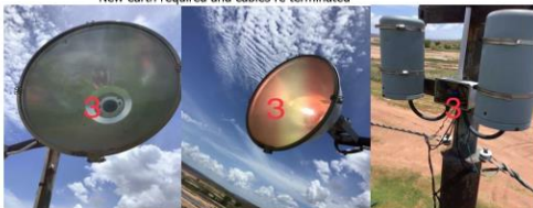
LIGHT TOWER 4 left light - faulty globe Right light - faulty ballast and globe New earth required and cables re terminated
