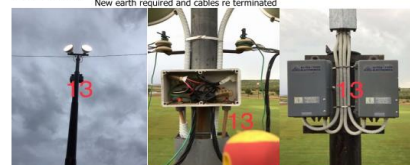
LIGHT TOWER 13 - Both sides of tower working fine New earth required and cables re terminated
