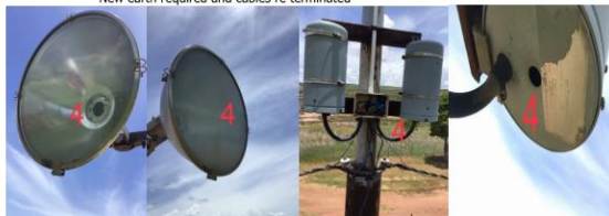
LIGHT TOWER 4 left light - faulty globe Right light - faulty ballast and globe New earth required and cables re terminated
