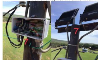
LIGHT TOWER 7 - LED lights both sides working fine New earth required and cables re terminated
