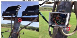
LIGHT TOWER 10 Left side - working fine LED Right side - faulty LED fitting New earth required and cables re terminated
