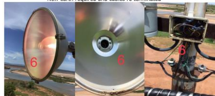
LIGHT TOWER 6 Left light - working fine Right light - faulty globe New earth required and cables re terminated
