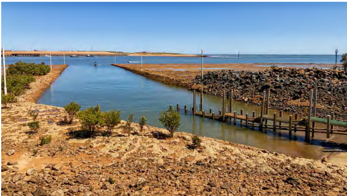
Figure 6-12 Example of a 'sheltered' inland boat ramp located in Port Hedland.
