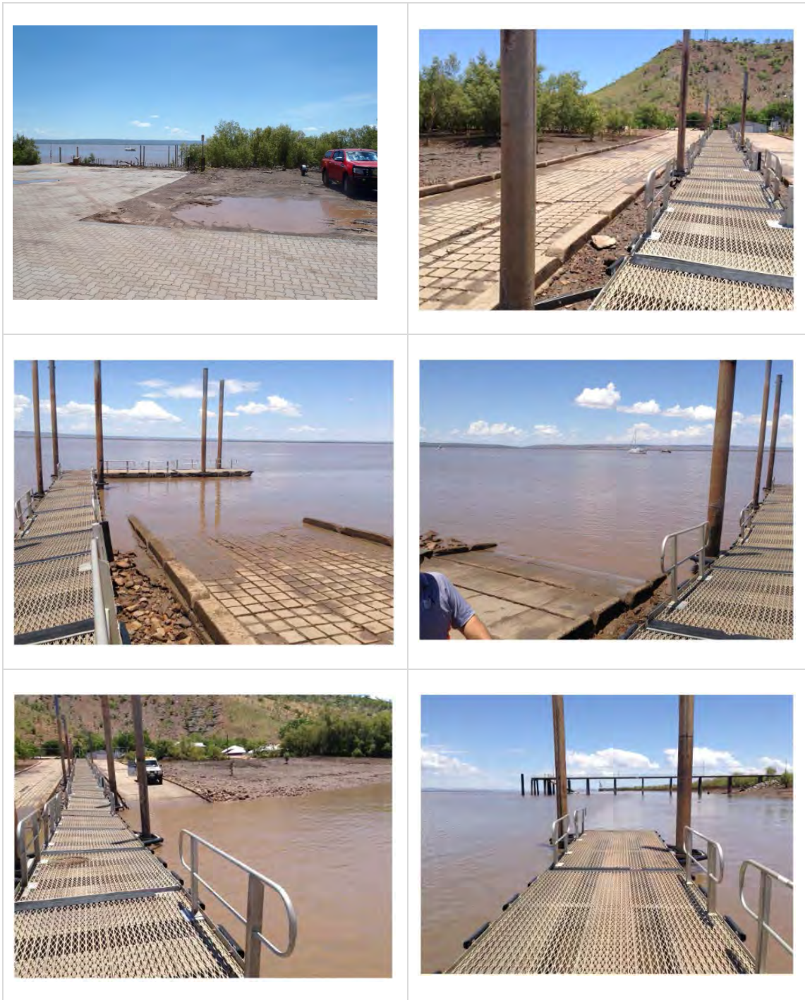
Figure 3-2 Photos of the Existing Wyndham Boat Launching Facility
