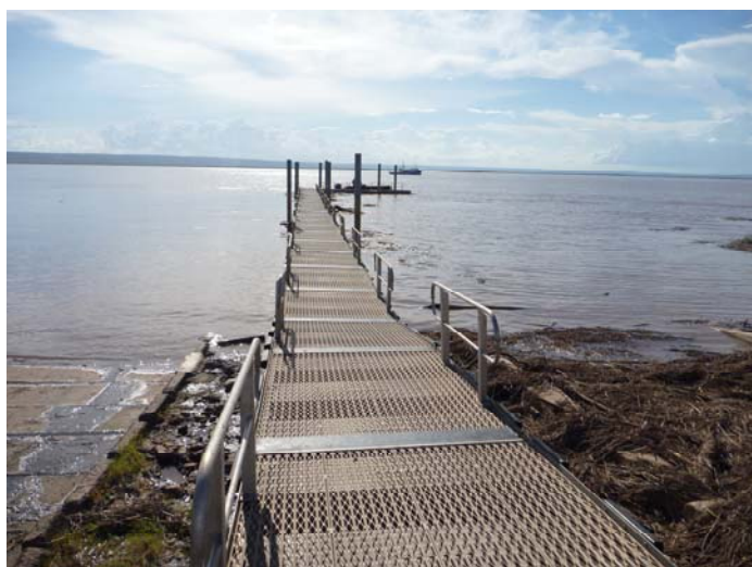
Photo 1: General view of structure
