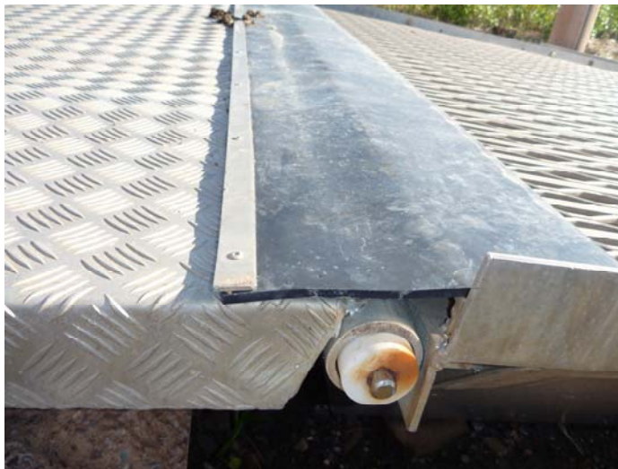
Photo 2: Hinge joining pontoon units with rubber cover strip
