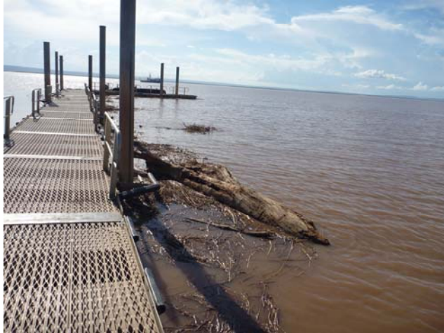
Photo 4: Debris caught on structure
