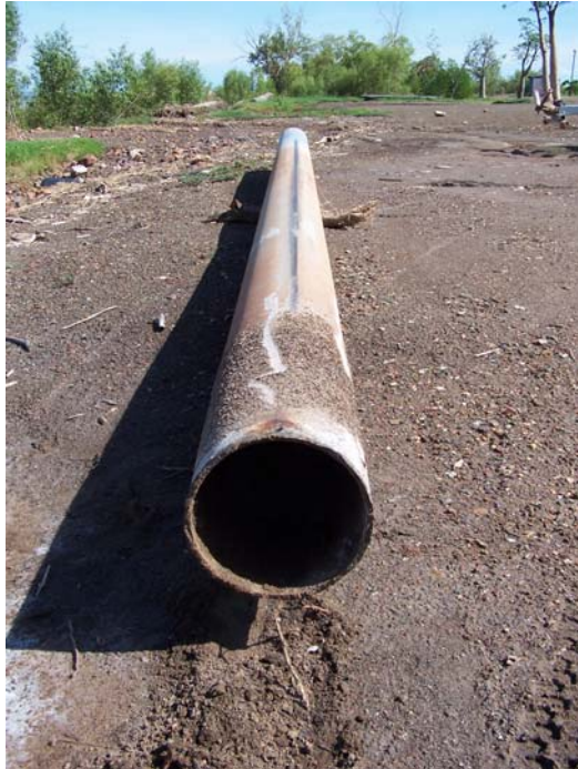
Photo 7: Broken pile (15 December 2010 failure)
