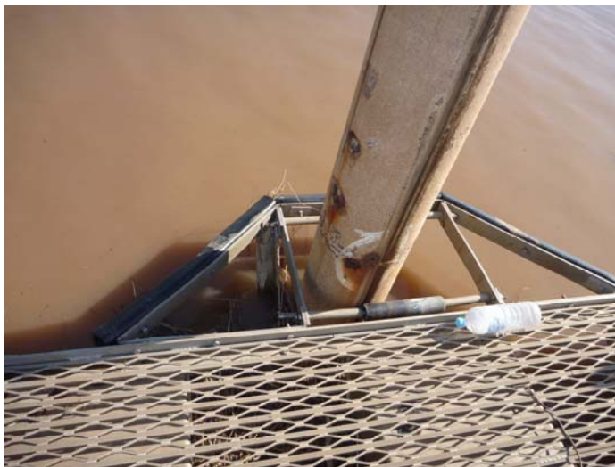
Photo 7: Corrosion on steel pile
