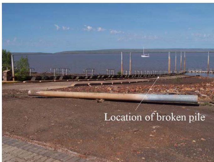
Photo 5: Broken pile (15 December 2010 failure)
