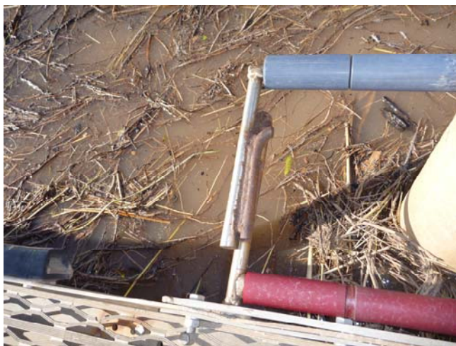
Photo 3: Pile Guide with repair in place
