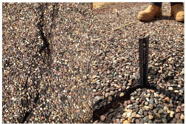
Where cracking is observed as increasing, a ruler was let drop into the crack to demonstrate penetration into base course. As the ruler is not flexible, it does not indicate true depth of cracking.
