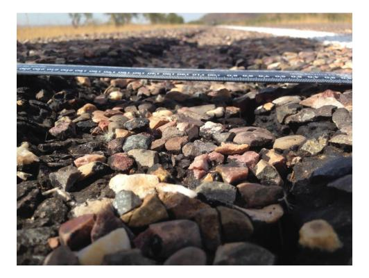
In some instances, cracking is splitting, with road material between the cracks sinking. This was demonstrated by placing a ruler over the span.
