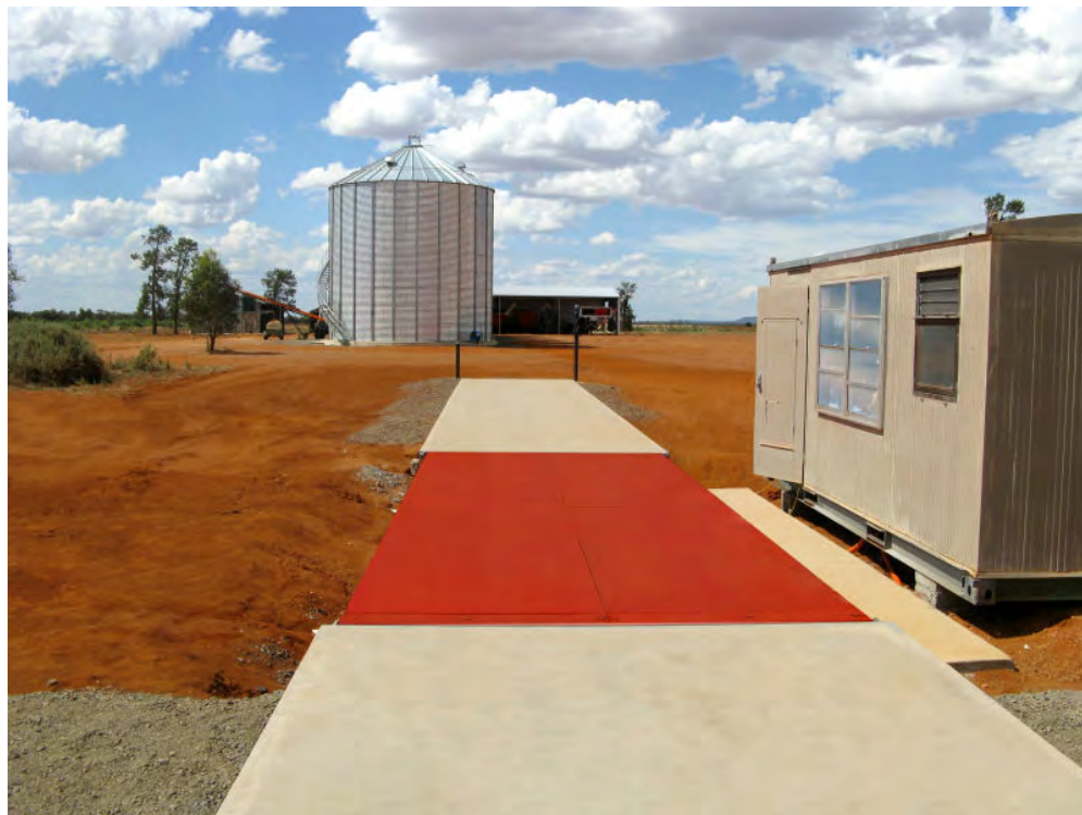
Figure 1 Steel relocatable weighbridge (12m) with concrete ramps
