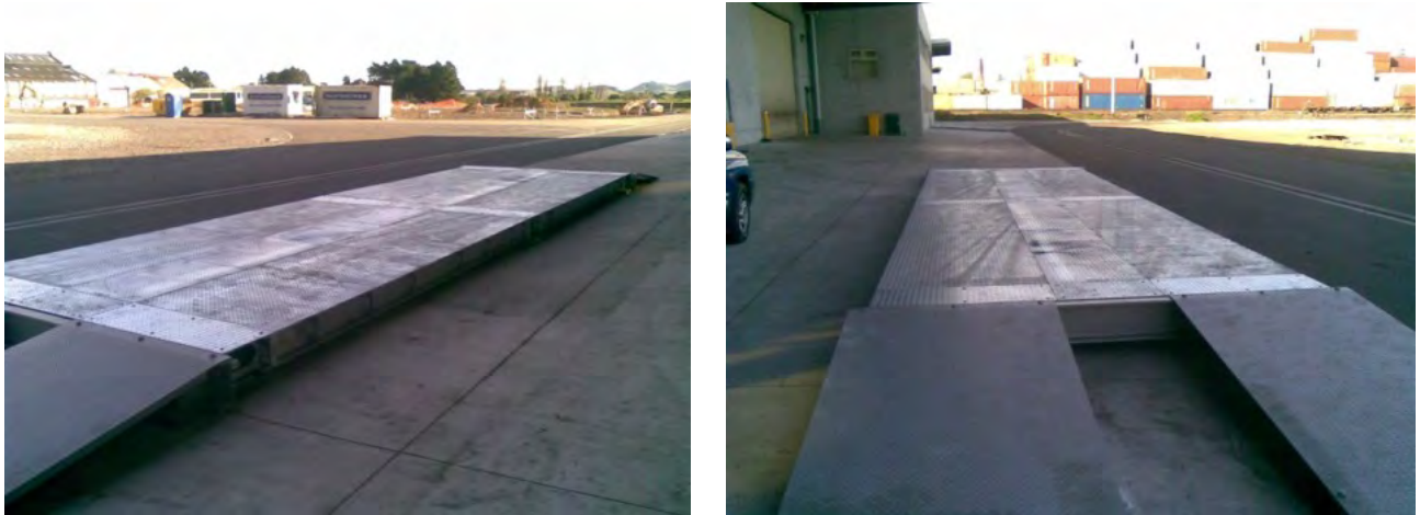
Figure 2 Steel relocatable weighbridge (12m) with steel ramps
