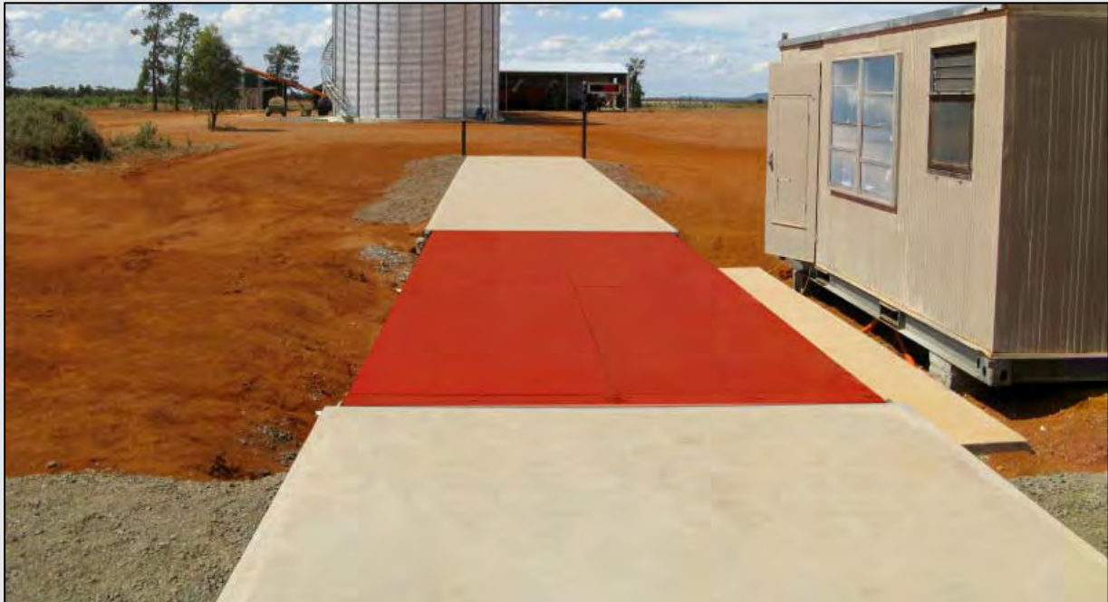
Figure 1 Example of a steel relocatable weighbridge (12m) with concrete ramps
